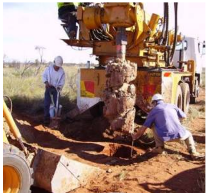
Drilling and sampling below the water table
